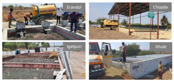
Figure 4: Sludge drying beds in Erandol, Igatpuri, Chopda and Dhule
