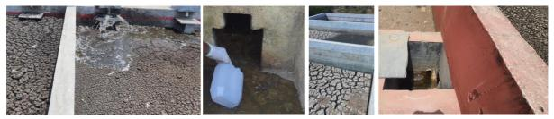
Figure 7: Collection of dried sludge at FSTPs in Erandol, Igatpuri, Chopda and Dhule (From left to right)
